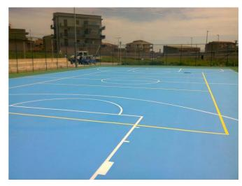
2. After the application of the mat, proceed with the application of the coating for the multi-purpose surfaces Floorgum Paint (see technical datasheet).
